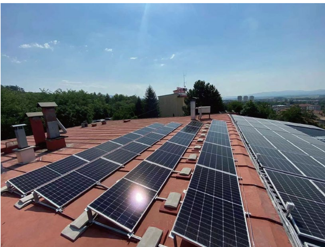
Ballasted Mounting-Bulgaria
